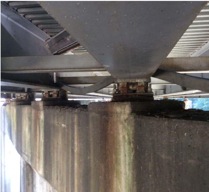
PHOTO 1 Description Bent 7 bearings have corrosion due to leaking joint seals. Common all bents.
