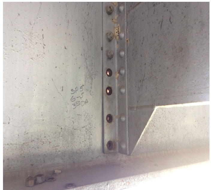
PHOTO 2 Description Span 5 beam 5 diaphragm 3 has four missing bolts.
